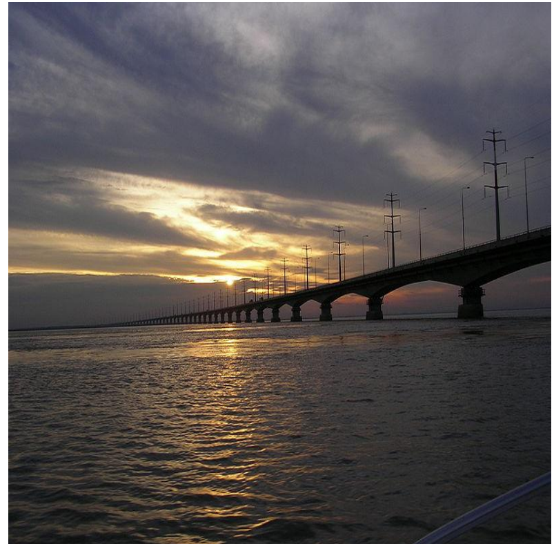
Jamuna Bridge, Bangladesh
